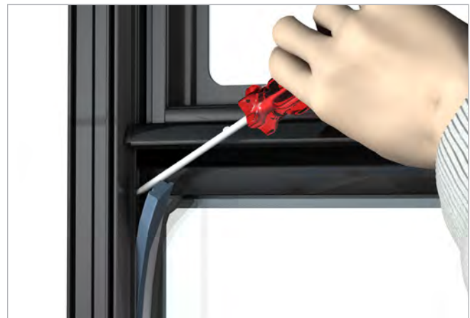
Figure 3 - Shield retainer rubber removal.
