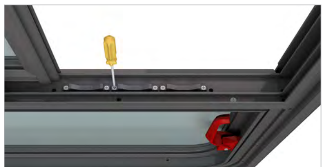
Figure 4 – Installing new strikes.
