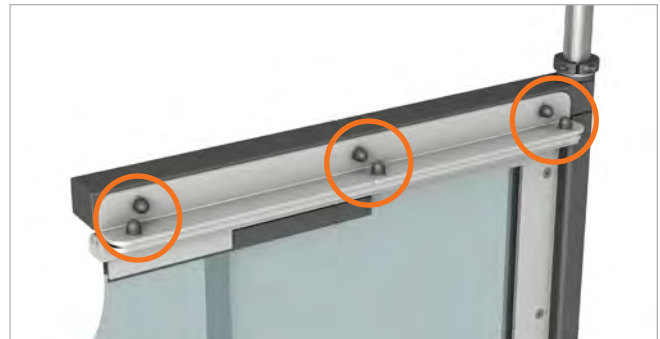
Figure 1 – Removal/replacement of plastic nut covers.
